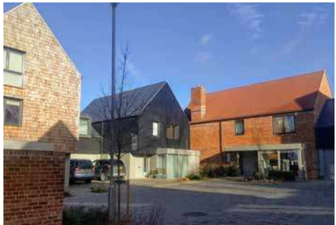
Figure 6.32 The Avenue, Saffron Walden. Representative example of a medium density layout arranged around courtyard blocks and streets
