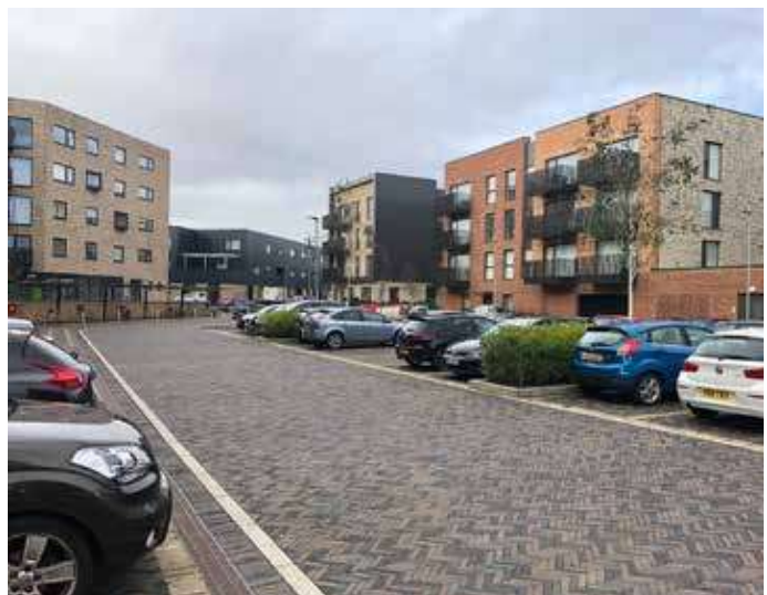
Figure 8.18: Clay Farm, Cambridge. Representative example of a well designed and enclosed landscaped perimeter parking courts
